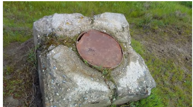
Photograph 6: Inactive water well near southern edge of the Subject Property.
