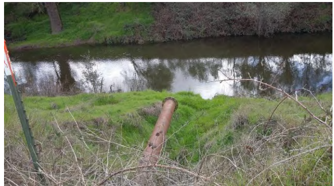
Photograph 18: Stormwater drain-pipe drains from the northern field to creek.
