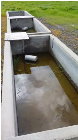
Photograph 11: Water trough on east side of Subject Property, north of well and AST.
